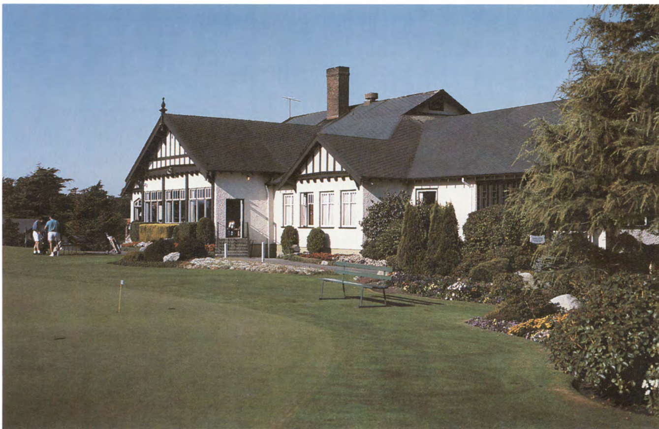
The Clubhouse before renovations began in September 1992. BOB TURNER
