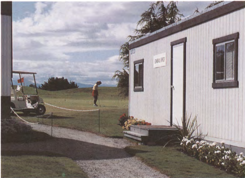
During renovations, the Clubhouse complex consisted of portable buildings. The photographer, thinking it was the construction camp, was astonished to see flower beds alongside the buildings. BOB TURNER
